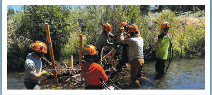
Building pole-assisted log structures (PALS).
